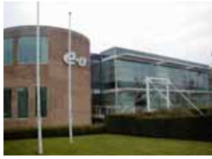
The modern main entrance/reception building
