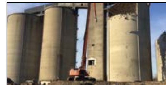
figure 25: Sproughton Sugar Beet Factory – demolition of silos
