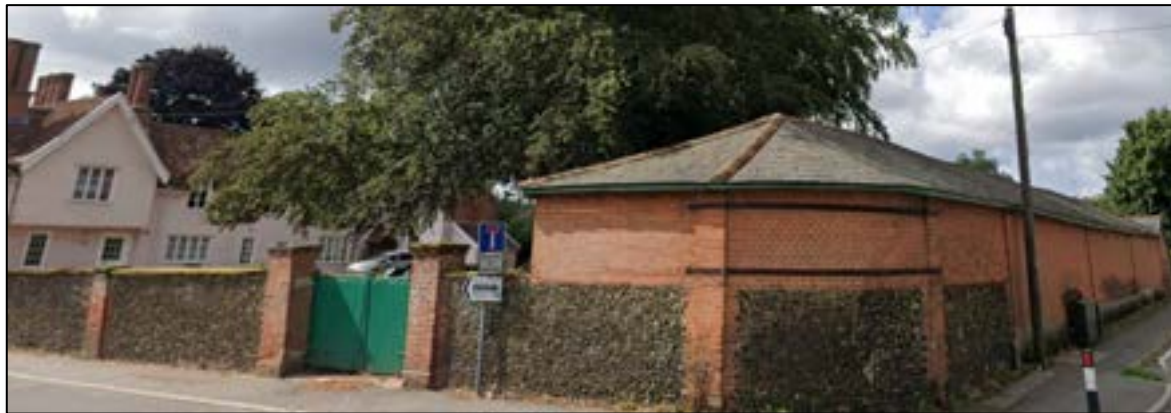
figure 103: Boundary Wall and outbuilding, 1-4 Church Close (facing Church Lane & Lower Street)
