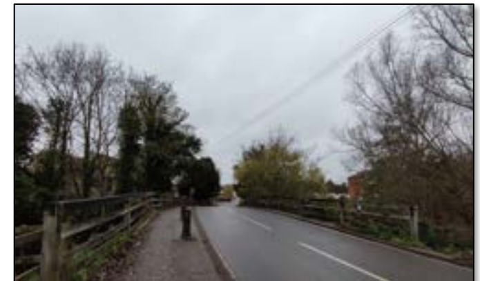
figure 77: View 3: Sproughton Bridge looking west
