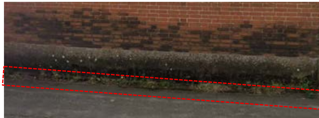
figure 150: Adjacent footway (weed strip)
