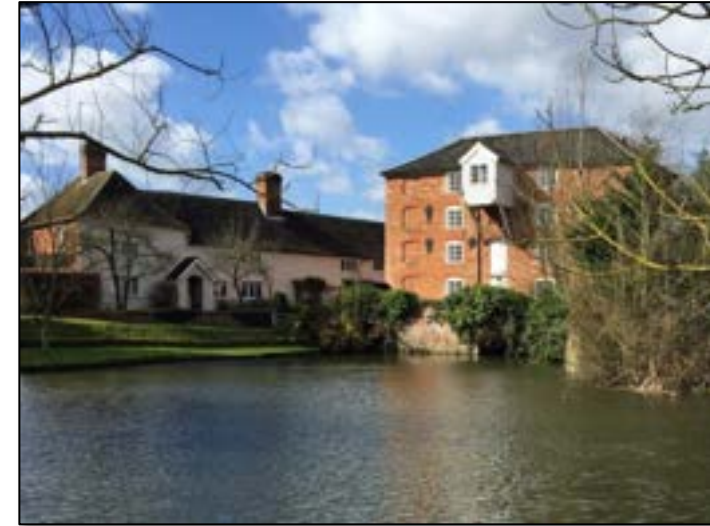
figure 106: Sproughton Water Mill (Grade II)
