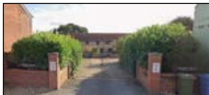
High Street – The Old Stables
