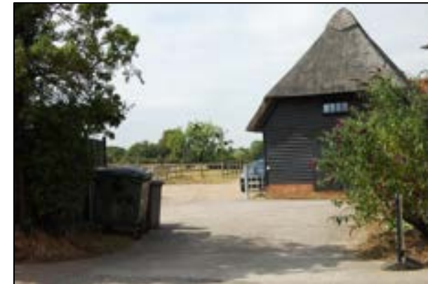
figure 82: View 7: Root Barn from Lower Street
