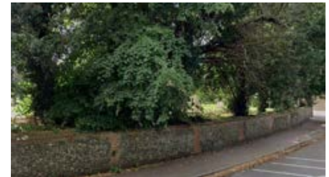
figure 105: Church Yard Wall and trees (facing Lower Street)
