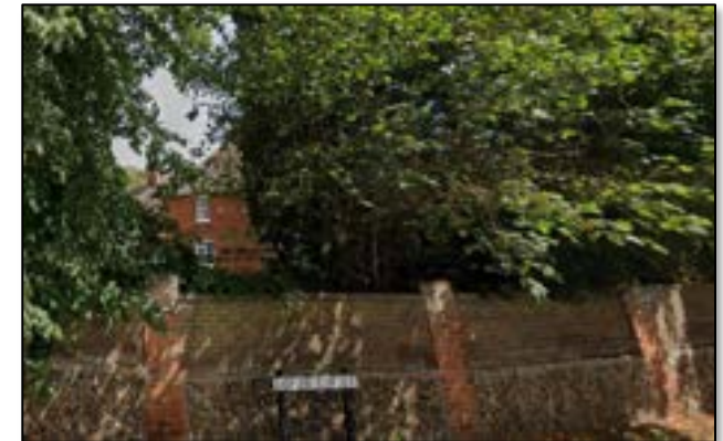
figure 104: Boundary Wall, Mill House (facing Lower Street)
