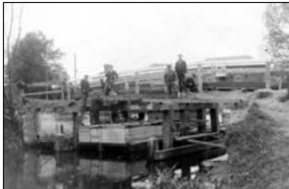
figure 96: Repairs to Sproughton Bridge 1906 David Kindred
