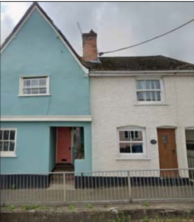
figure 122: Municipal Safety barrier Lower Street [visually unsympathetic]
