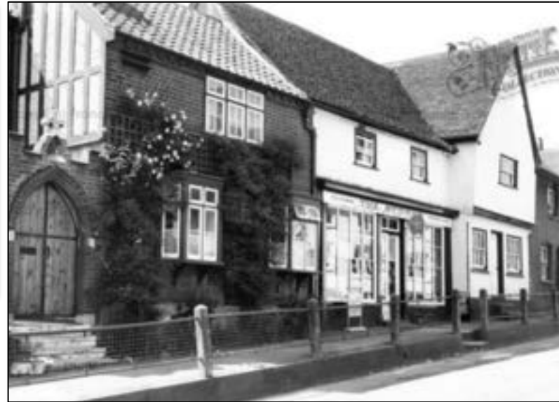
figure 147: Railings 1965 [ visually these look sympathetic ]
