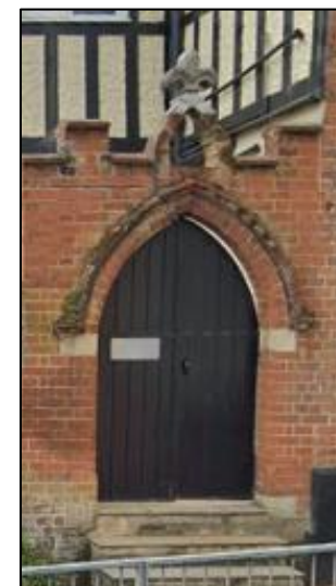
figure 117: Street gate to Rectory Cottage
