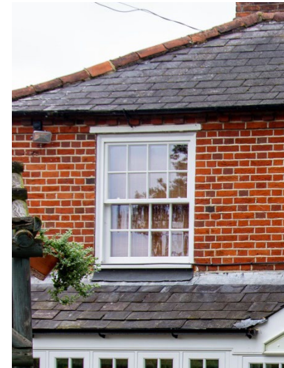
Sash window with glazing bars
