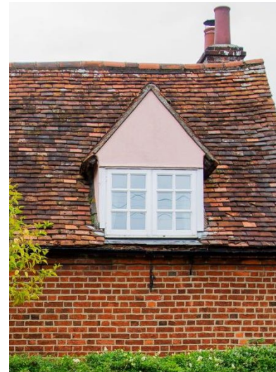
Casement window with glazing bars
