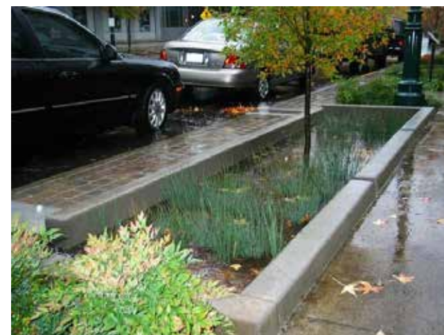
Figure 109: Example of sustainable drainage incorporated into the street scene.
