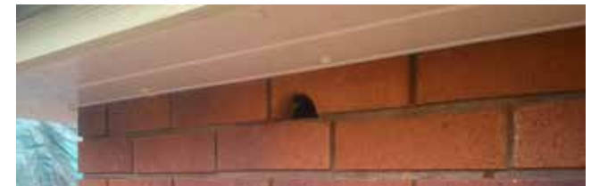
Figure 120: Example of a swift brick under an eave.
