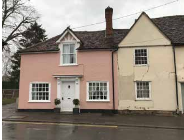
Figure 43: House with windows with double-hung sashes, glazing bars and white, flush cased frames.
