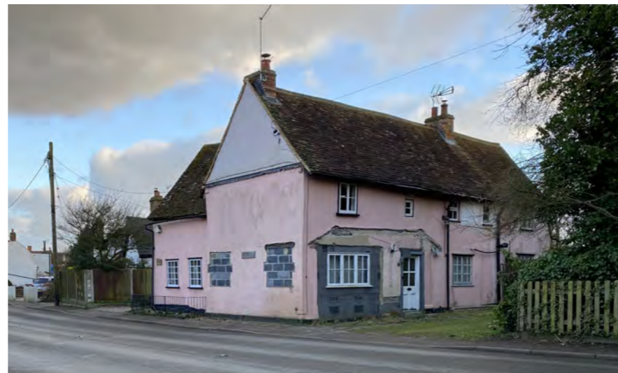
Figure 244: Gasgoines/Chaplains Cottage—listed building at risk.
