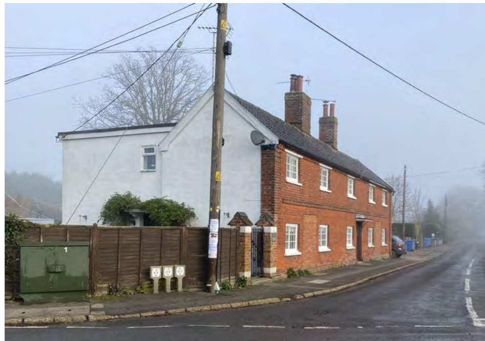
Figure 206: The positive contributor cottages at 1-3 Gandish Road somewhat slighted by unsightly standardised utilities installations, and a somewhat over sized rear extension.
