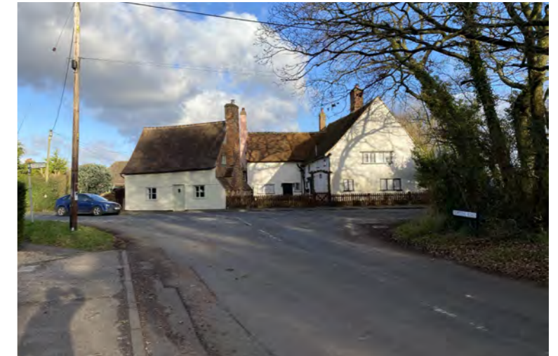
Figure 140: View along Quinton Street past the Box Iron to Quintons House and Cottage which terminate the view.
