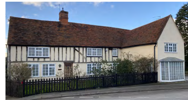
Figure 12123: Stuarts formerly known as 'Tarbin & Jessops' and above the bay window and northern elevation when in use as a shop from the mid 20th century above (History Group: East Bergholt Back in time group)
