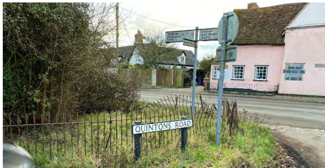
Figure 241: The southern apex of Quintons Corner, damaged railings, somewhat cluttered collection of signs, the background greenery is a positive screen to post enclosure development but the condition of this area is poor. The listed building 'Gascoigne's' is visible in the background and is on the Heritage at Risk Register.
