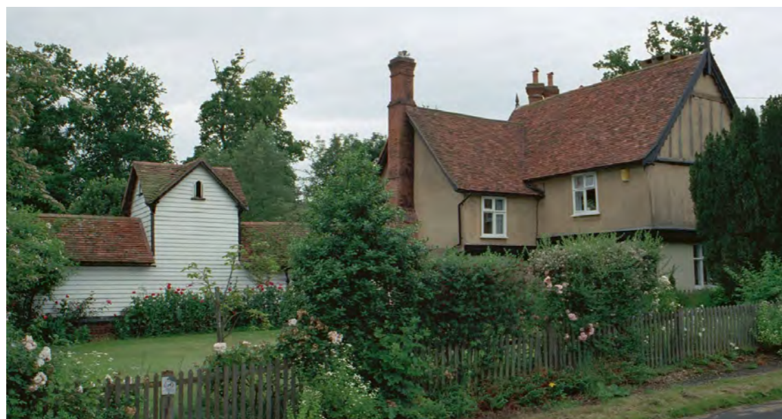
Figure 193: Claycotts and its associated outbuilding on the left. Rendered timber framing and the highest grade listed building in this sub area at II* (image: EBS)
