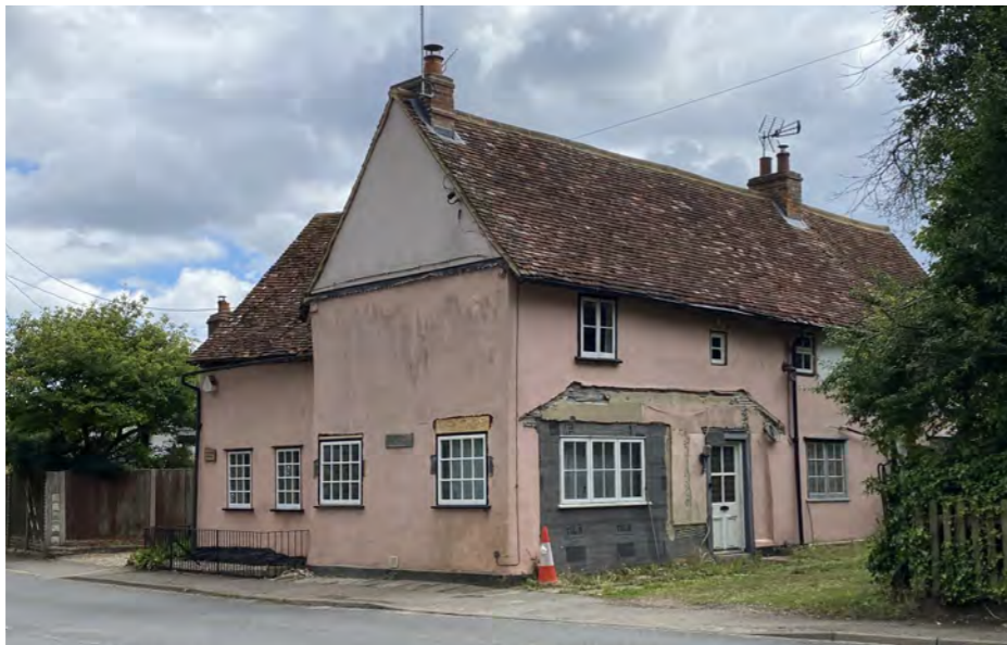
Figure 148: Chaplains and Gascoignes Cottage, a listed building in poor condition, summer 2025
